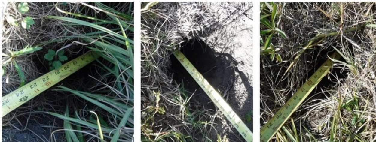
Figure 8. Forage Holes and Depths Observed on External Slopes of the Surface Impoundment System and Pump Back Ponds
