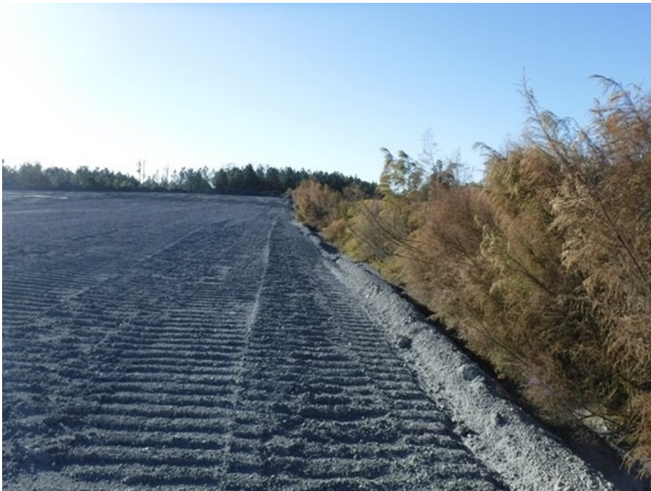
Figure 12. Grading Along Western Side of Cell 1
